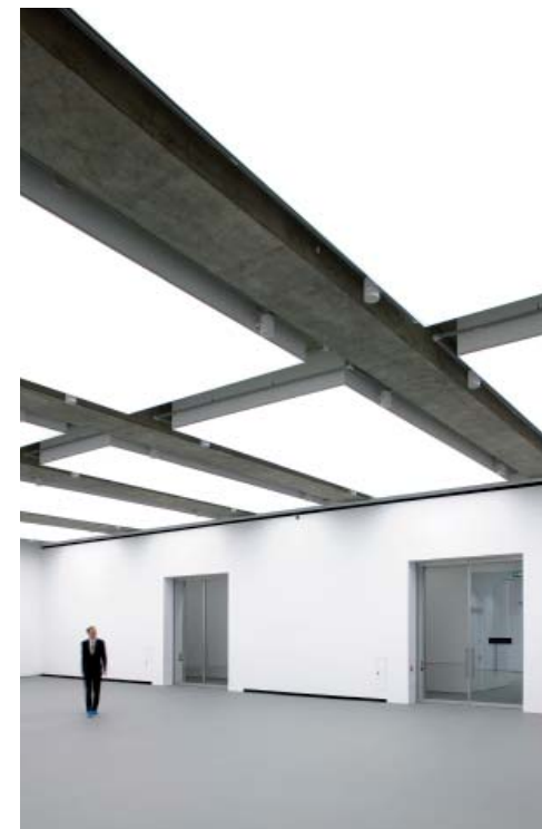
Light boxes provide controlled artificial light to the galleries in the new Towner gallery in Eastbourne, UK
